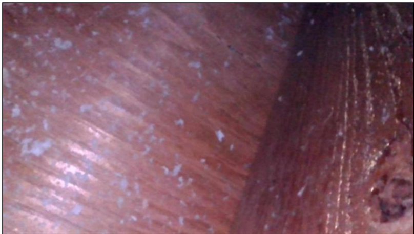
1.0 Concealed, non-moisture damaged wood framing, shown for comparison purposes; viewed from borescope camera. This is what we should see when there's no damage.
