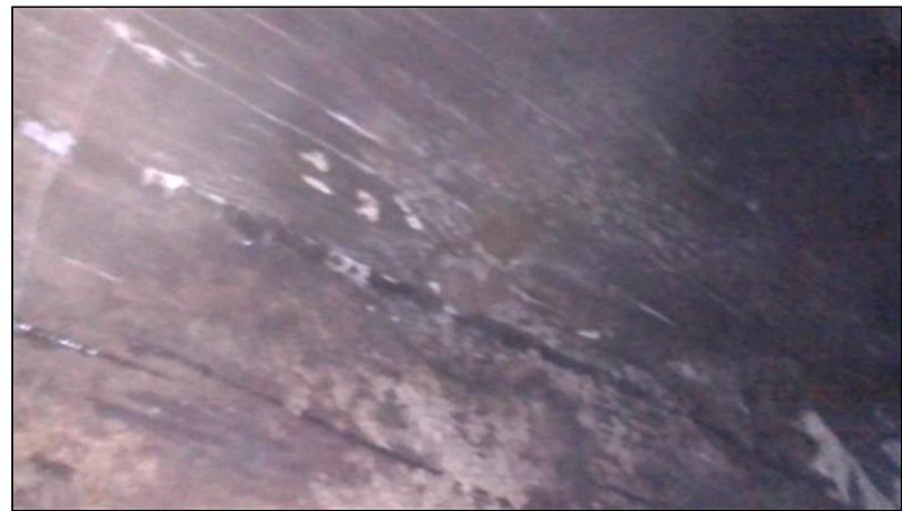
1.0 Concealed, Moisture damaged wood framing; viewed from borescope camera
