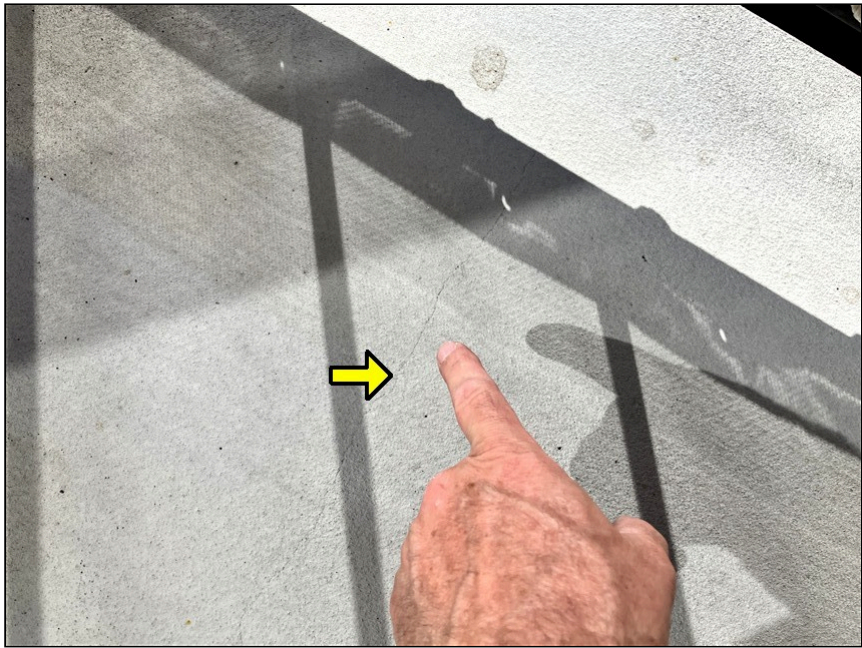
2.0 Cracks at fiberglass traffic coating
