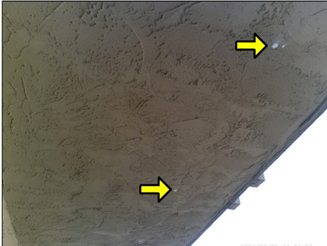
9.9 Tight fitting plugs were installed to repair all locations where holes were drilled.
