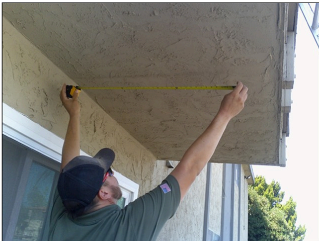
9.3 Measuring for proper location of holes to be drilled
