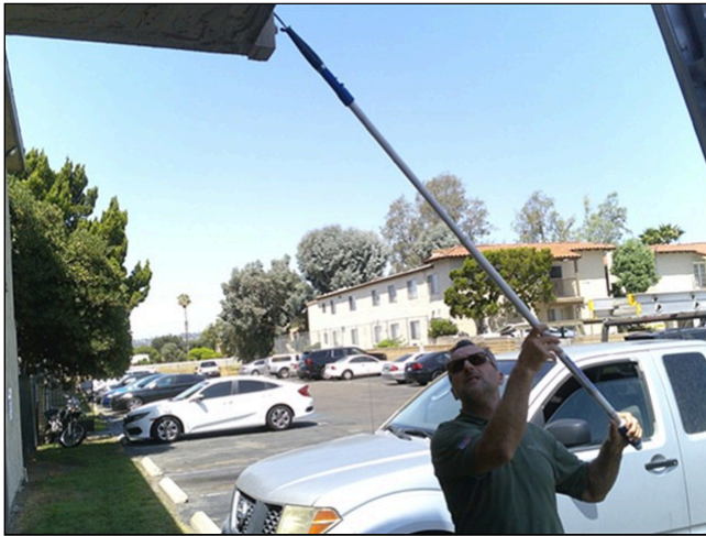
9.8 Inspector probing exposed wooden components for defects
