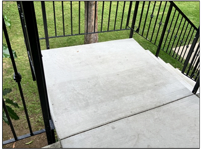
The concrete walking surfaces serving serving units 20 & 33 landings were inspected and deemed to be in good condition/ no defects
