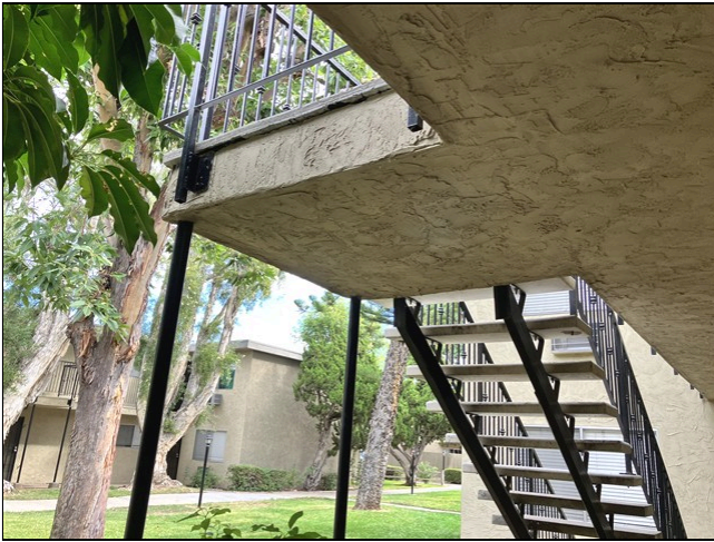
The landings serving units 20 & 33 were inspected and deemed to be in good condition/ no defects
